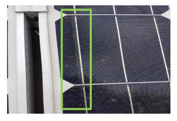
Visible cell damage on the module with an Earth Fault was easily detected with Tigo's module-level monitoring.
